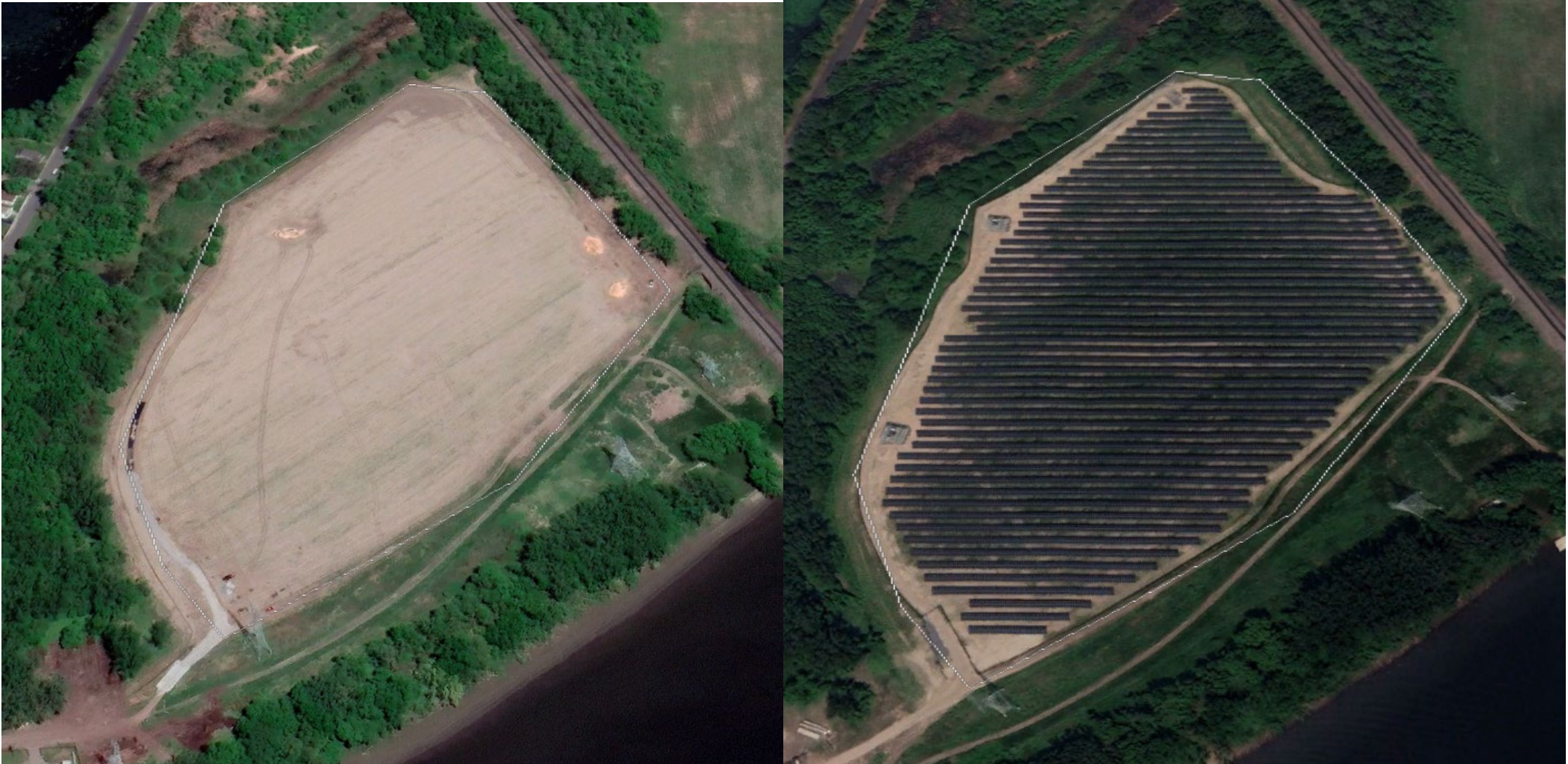
6MW solar arrays near Mohawk River & Albany installed in 2021 (left: 5/2020; right: 5/2021)
